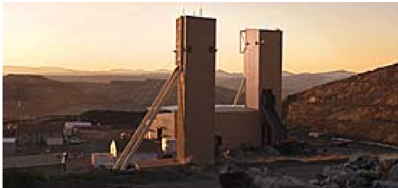
Newmont's Leeville Underground Project in northern Eureka County. Newmont is one of the county's principal taxpayers Photo courtesy of Newmont Mining Corp.
