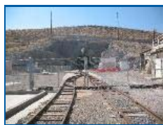
A gate on a security fence blocks the north entrance to the 5-mile tunnel that loops into Yucca Mountain, located 100 miles northwest of Las Vegas. The Department of Energy closed the exploratory tunnel earlier this year for safety concerns following funding cutbacks that eliminated staffing and forced officials to shut off ventilation and lights.
