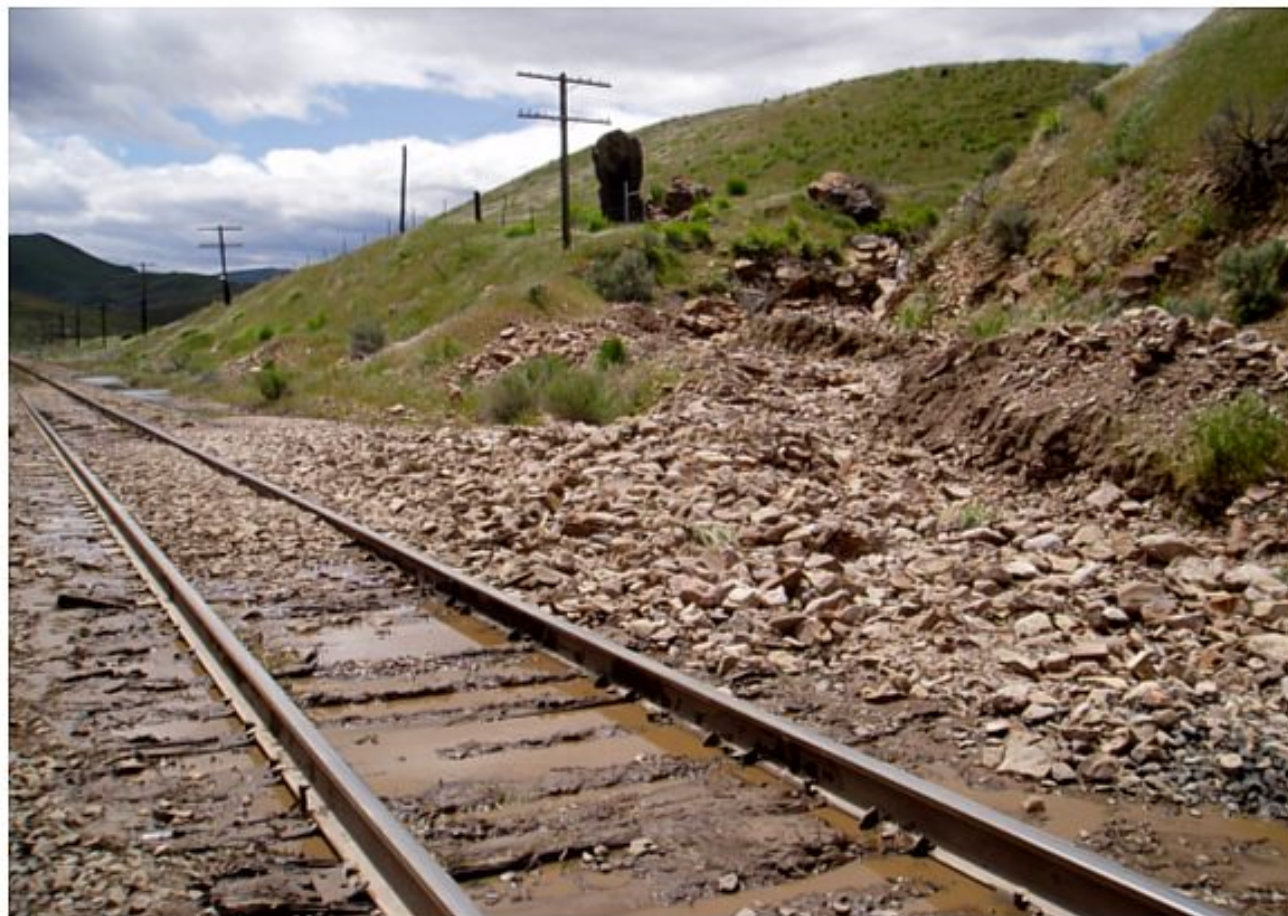
10: Rockslide and muddy tracks, north of Palisade townsite on westbound track.
