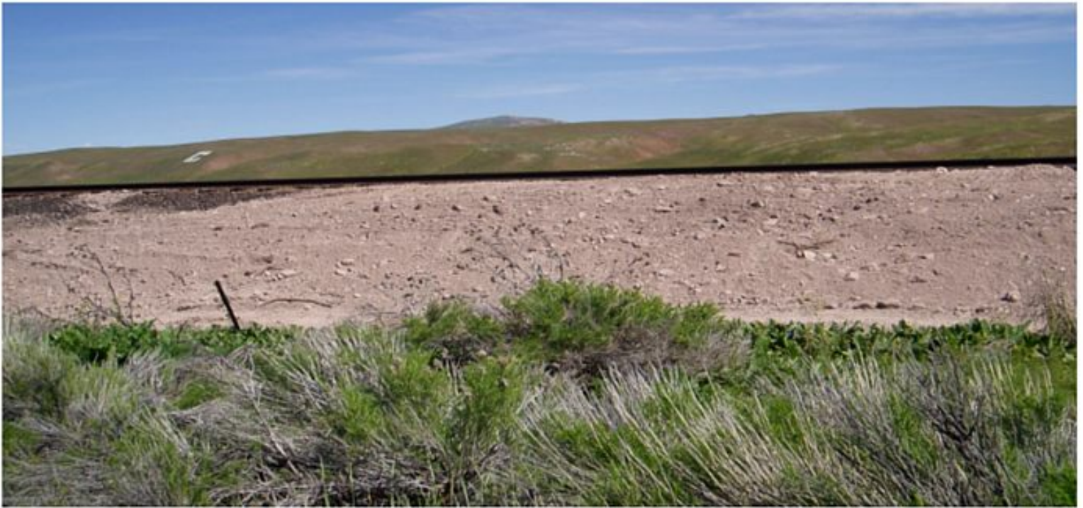
7: Opposite side of the rip-rap (above). Fresh dirt was laid on this side because the flood water had apparently saturated the existing dirt under the tracks.
