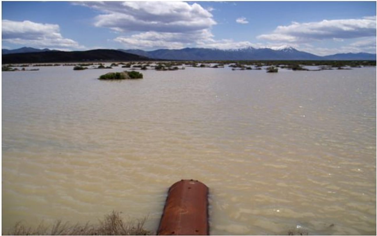
5: At the east end of McDaniel Way, where the culvert is running under the Eureka County Road. The flooding is within the potential "Carlin Spur" rail corridor area.
