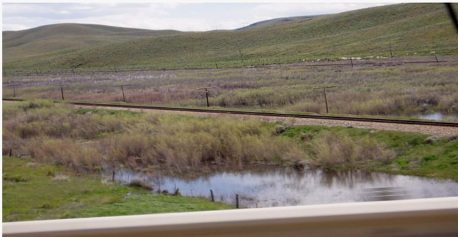
8: Standing floodwater on both sides of the track. Picture was taken from I-80, looking south, where the highway goes over both rail lines at the TS overpass.
