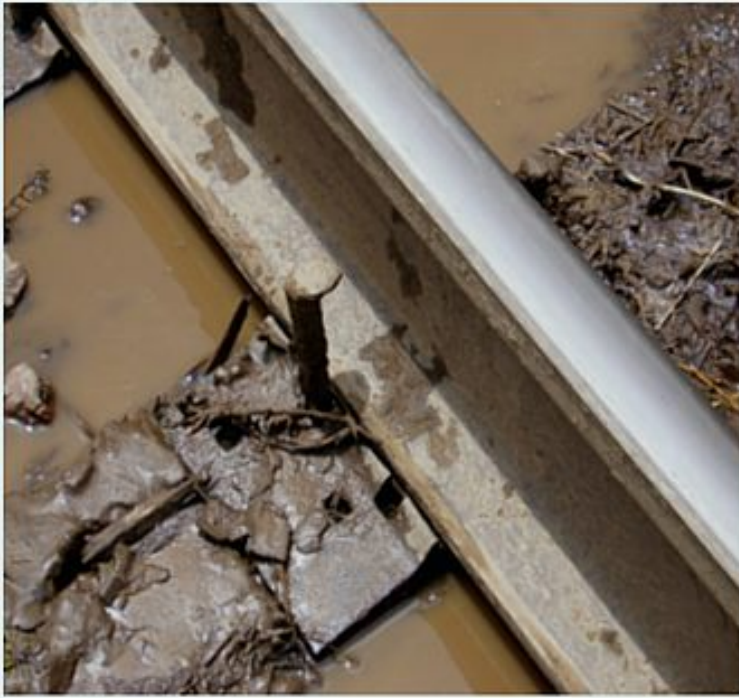
11: Close-up of a raised rail-spike from picture 10. 12: Rockslide and ponded flood waters. Opposite view of picture 10.
