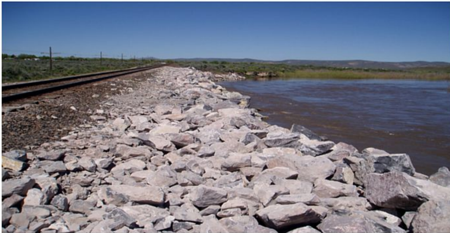
6: Flood waters from the Humboldt River were turned away at the bank of this rip-rap just east of the Carlin Bridge. The rip-rap had been placed by railroad workers May 19, 2005.
